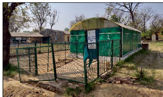
Covered with Sandwich Foam Plastic Panels
